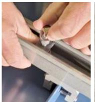
5. Set the second rail with the attached satellite bracket, over the seams so the other side of the bracket can be attached to the already installed first rail. Use the included spring channel nuts to attached the satellite mounting base to the first installed rail, leaving the bolts loose for now. Mount and tighten the Roof Clamp top bolts and set screws to 90 inch pounds. Equally tighten the channel spring nut bolts holding the satellite mounting base.
