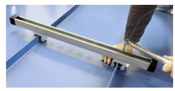
4. Attach the base of the satellite mounting bracket to the lower rail (not yet installed) using the supplied channel nuts and bolts. The channel nuts are inserted spring first into the Unistrut and locked into place by twisting clockwise. Hold channel nut while threading bolt through your satellite mounting base into the spring nuts. Leave bolts loose until the second rail is attached to the seams.
